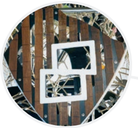
Totally twisted: facade elements overhead
