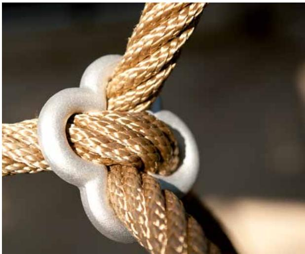
After safety rules were established for playgrounds, finger pinch points were also defined. Openings of  $> 8$  mm can't be prevented in all round ring applications. If rope lines of the same size are looped, the cloverleaf ring shape is required in order to avoid gaps.
